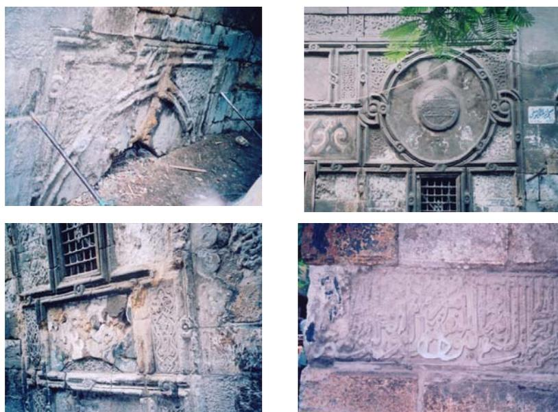
**Fig. (1)** Photos of Azbak limestone ornaments showing erosion, efflorescence of salts, discoloration, chipping and disintegration between grains.
