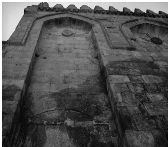
Fig. 5. A common characteristic of the mausoleum and most monuments built in Fatimid Cairo city; the big dark spots of humid aspect.
